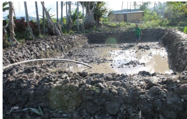
Hand-dug fish pond nearing completion
