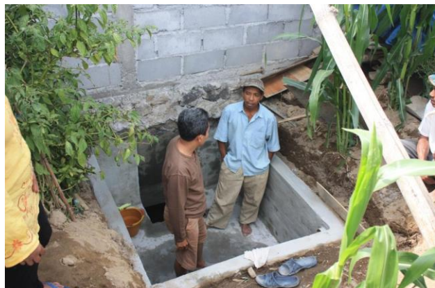
Concrete sump built for animal waste in Indonesia
